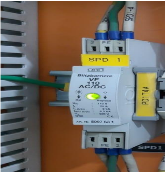
Fig. 1 Surge Protection Device Class D, 110 V AC
