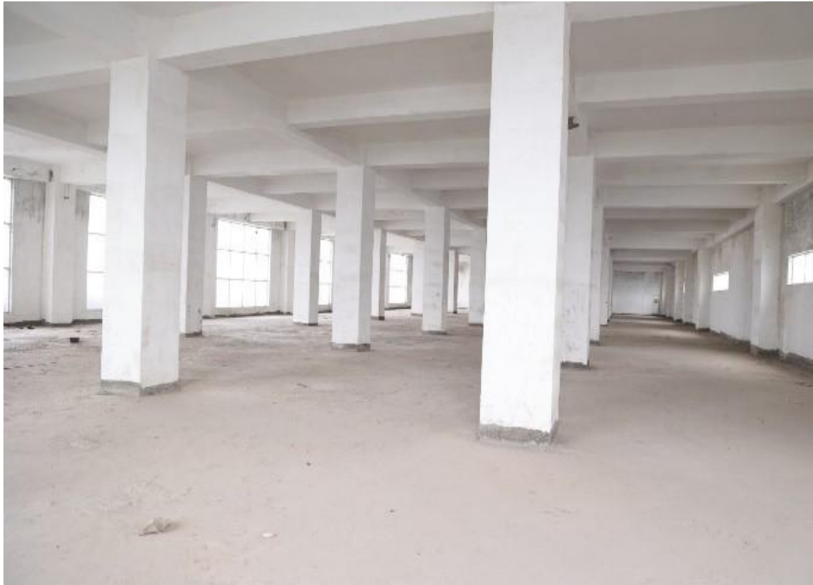
Site Photograph of offered commercial space with tentative area
