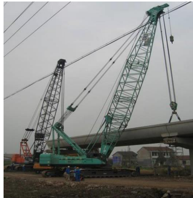
Figure 1: Placing full precast span (with crane)
