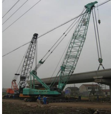
Figure 1: Placing full precast span (with crane)
