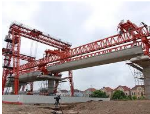
Figure 2: Placing full precast span (with launching girder)
