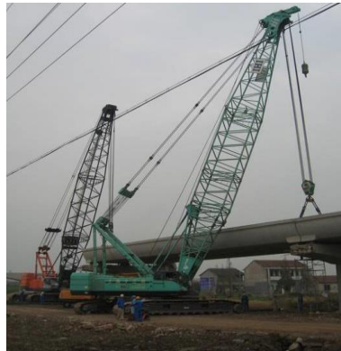
Figure 1: Placing full precast span (with crane)
