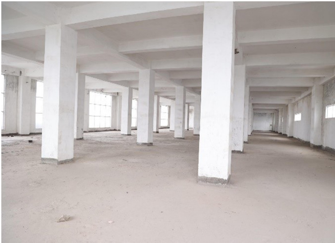
Site Photograph of offered commercial space with tentative area
